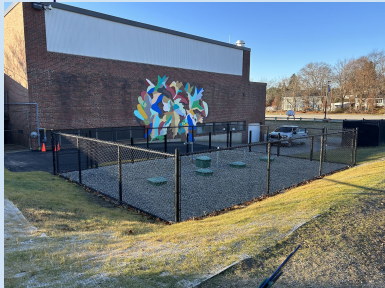
Completed conversion from oil to propane at Swanson Road Intermediate School
